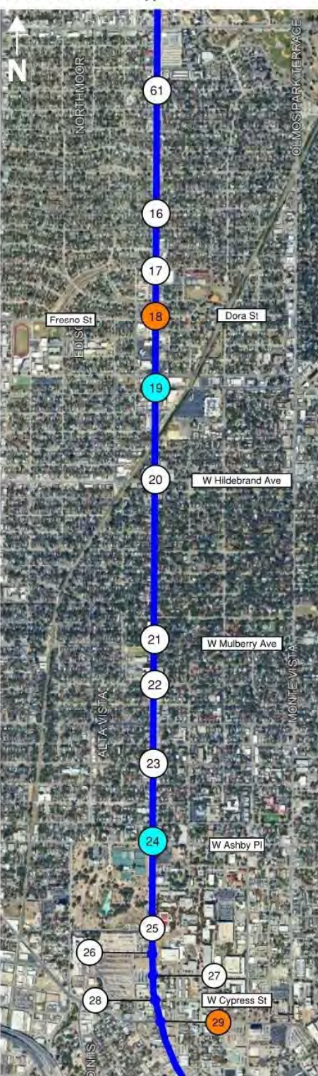
San Pedro Ave at Basse to San Pedro Ave at Cypress
